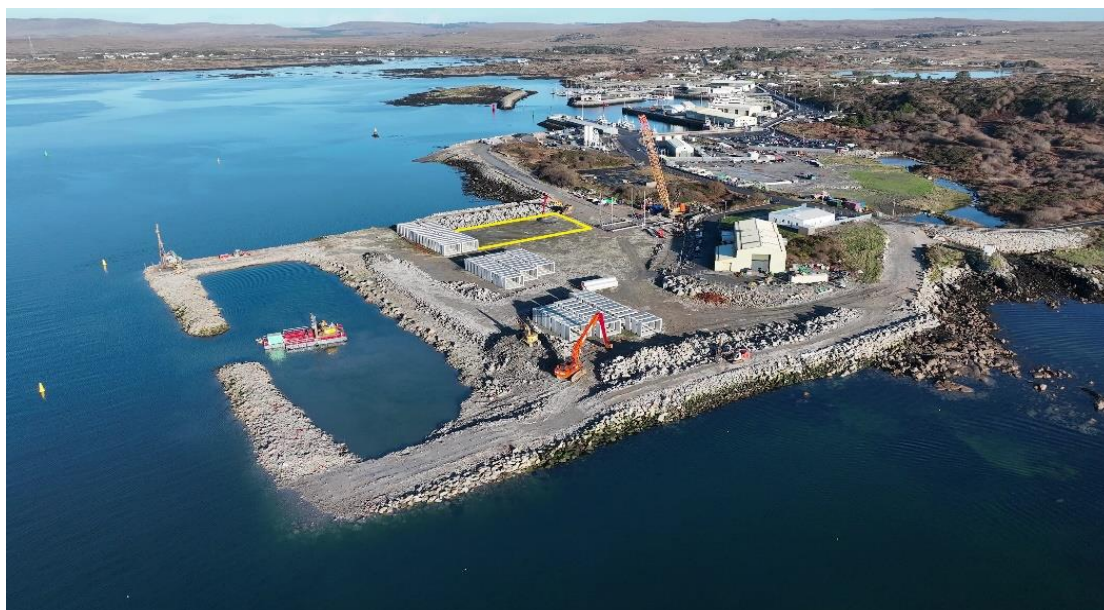
Plate 2: Drone image showing development of breakwater adjacent to the berthing circle. Dredge material designated placement area (yellow box).
