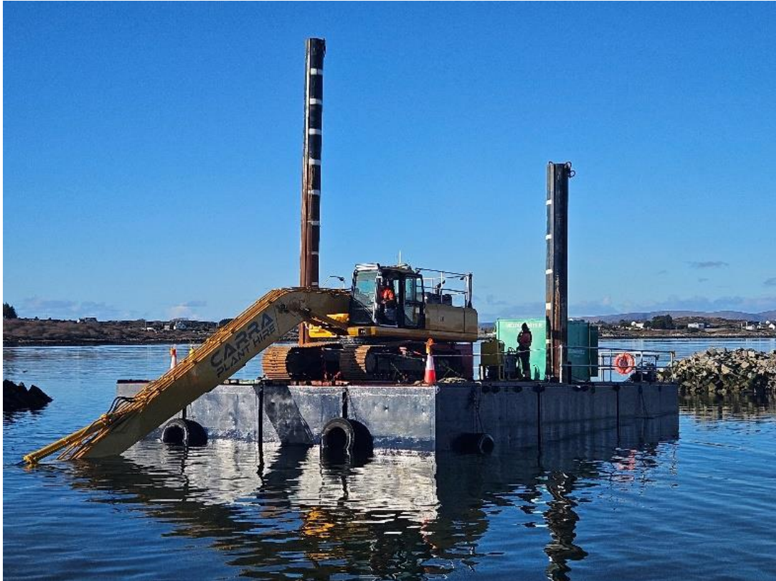
Plate 3: The dredging plant comprised a long-reach excavator mounted on to pontoon barge.
