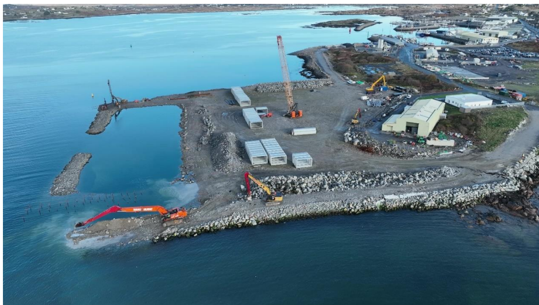
Plate 1: Drone image showing development of breakwater adjacent to the berthing circle.
